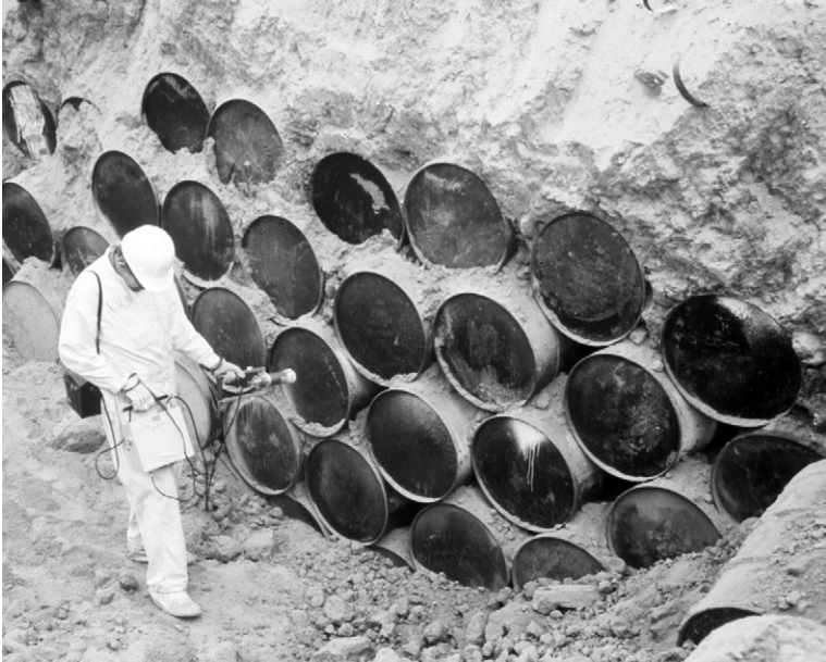
Figure 10.2 Worker checking buried low-level waste for radioactive leakage.
