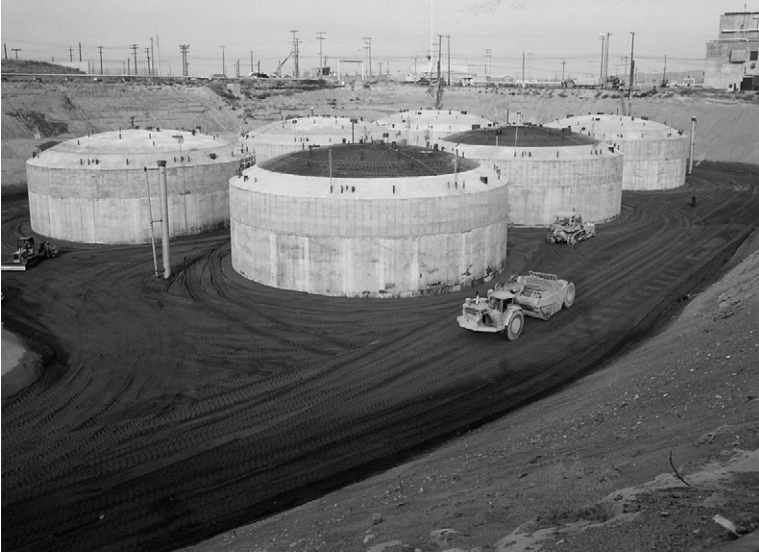
Figure 5.4 Hanford double-shell tanks under construction in 1978.
