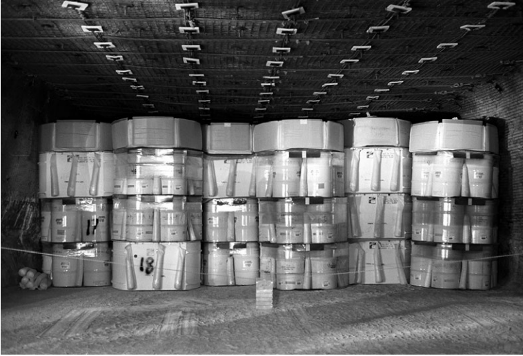
Figure 11.1 Transuranic waste containers emplaced at WIPP.
