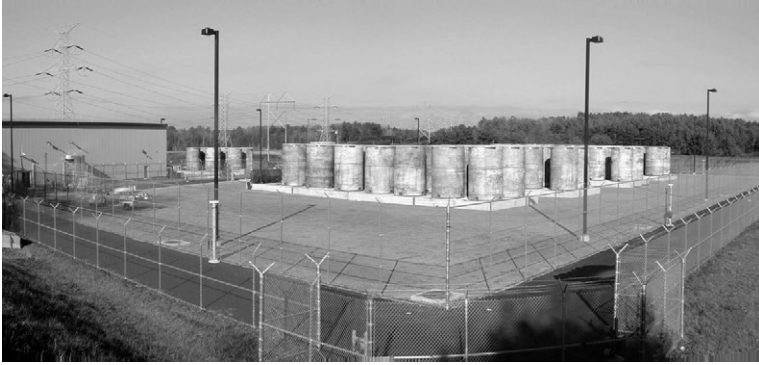
Figure 8.1 Dry cask storage at decommissioned Maine Yankee site. Courtesy Maine Yankee.
