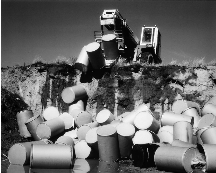
Figure 10.1 Cardboard waste drums randomly dumped into trenches.
