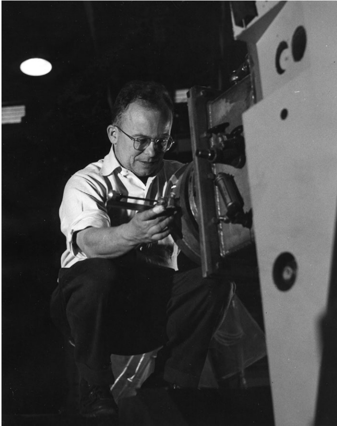
Figure 5.6 Wolfgang Panofsky adjusting an analyzing magnet used in meson experiments performed with the 1-Bev linear electron accelerator at the High Energy Physics Lab, Stanford, CA, 1959.
