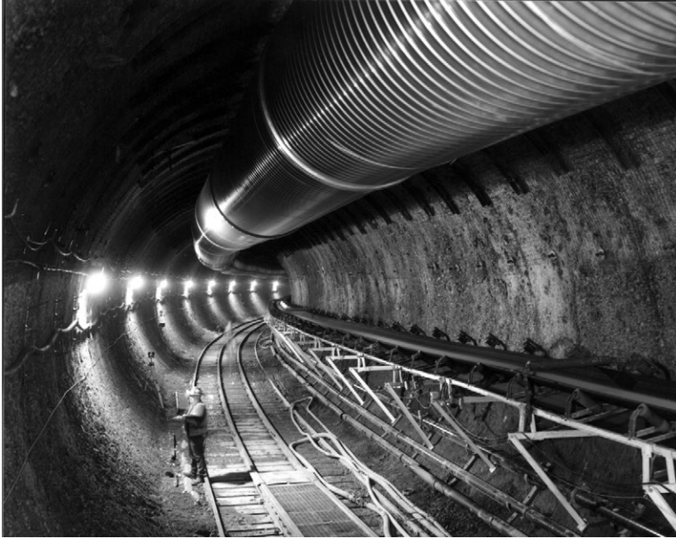
Figure 17.2 Exploratory Study Facility at Yucca Mountain.
