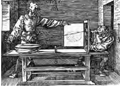
Figure 1 An artist using Dürer's perspective machine.
