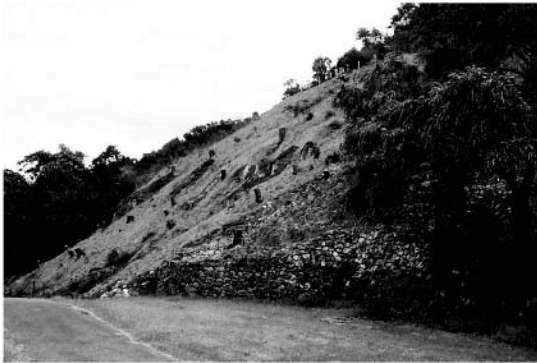
Fig. 11.2. Slope and Lower Walkway at Kings Park ©Survey Review: Gordon and Lichti (2004)
