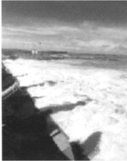
Figure 10. Operation of the VBAC Q=28.000 \text{ m}^3/\text{s} .
