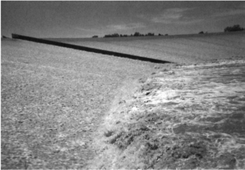
Figure 1. Air entrainment at Chinchilla weir (Australia)—Note self-aeration down chute and in hydraulic jump (foreground)—The beige colour of water is caused by three-phase mixing (air, water & sediment).
