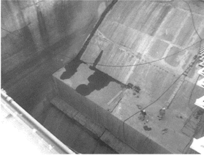
Figure 11. VBP: construction of the deflectors.
