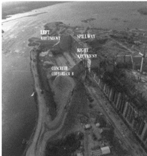
Figure 2. Aerial photograph of Caruachi Dam (Abutment details).
