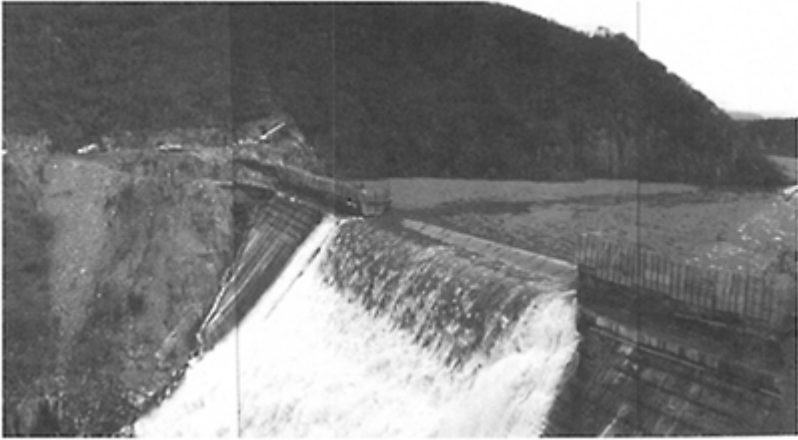
Figure 4. Skimming flow down Trigomil stepped spillway (Mexico): Q_w=1,017 \text{ m}^3/\text{s} , chute width: 75 m (Courtesy of Drs Sanchez-Briebesca and Gonzales-Villareal).
