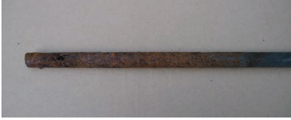
FIGURE 7.6 Uniform corrosion on a steel tube.
