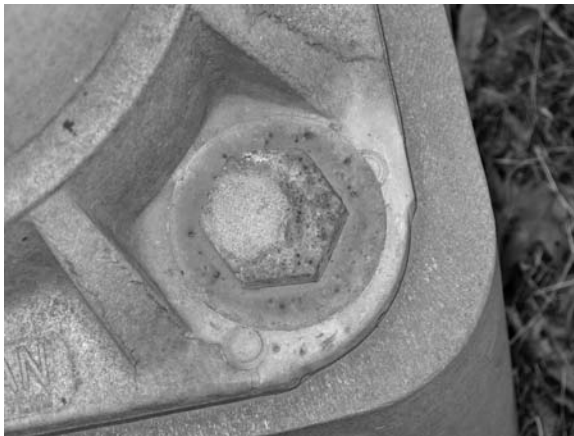
FIGURE 4.20 (See color insert following p. 142.) Localized corrosion.
