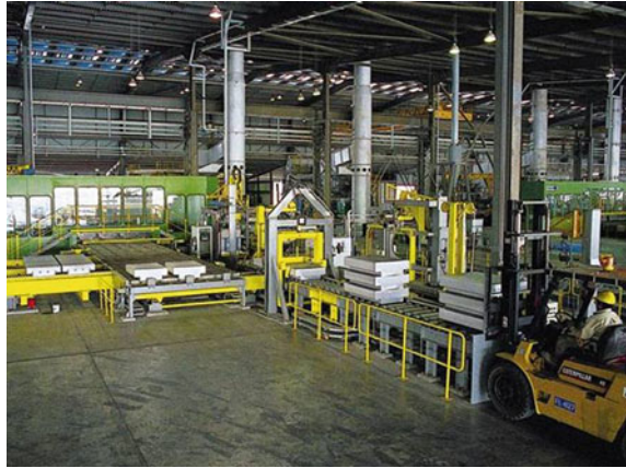
Fig. 20.16 Inside the T-Bar cast house (Courtesy: Hertwich Engineering)
