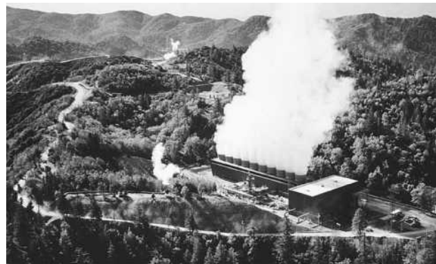
Located in Sonoma and Lake Counties in Calif., the geysers complex produces over 900,000 kW of electricity using steam from geothermal wells 7,000 to 10,000 feet below the surface. (U.S. Department of Energy)
