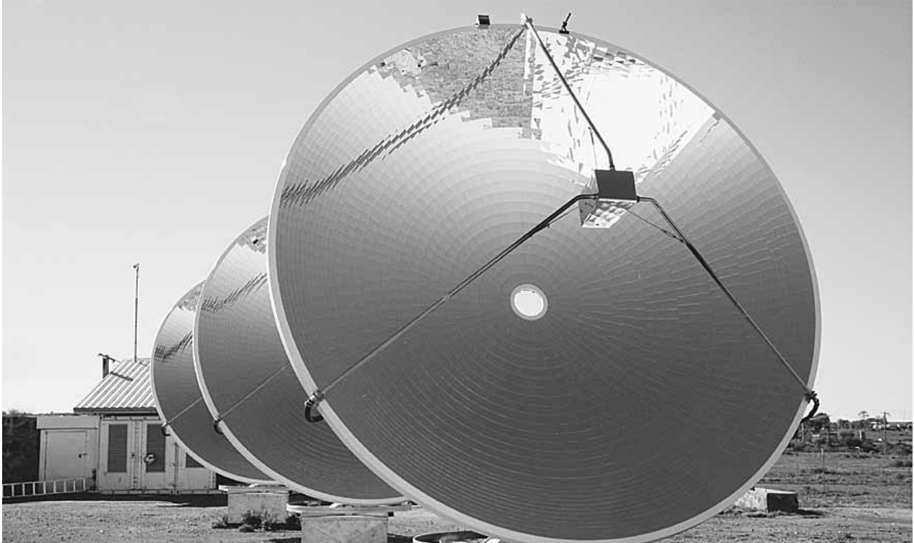
Parabolic solar energy concentrating dishes sit in a row at the power station at White Cliffs, Australia. The plant, operated by Solar Research Corp. of Melbourne, is Australia's first experimental solar station. (Corbis Corporation)
