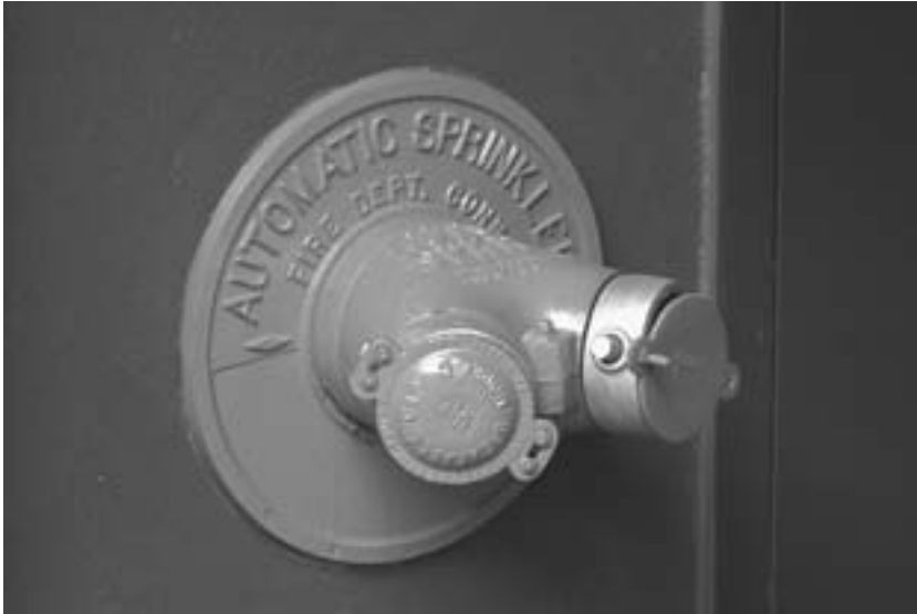
FIGURE 9.7 Sprinkler-system connection
