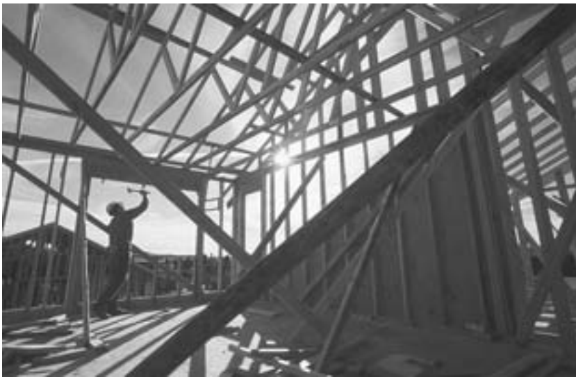
FIGURE 5.2 Wood-frame construction
