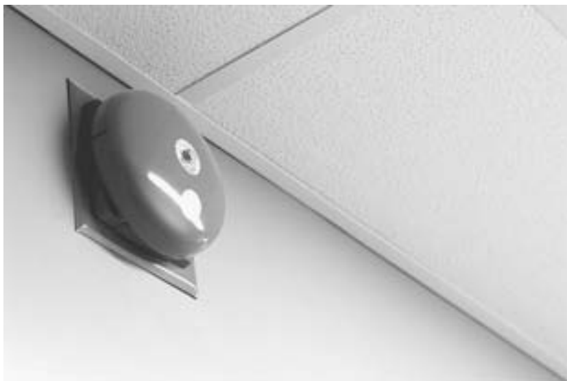
FIGURE 8.3 Fire alarm
