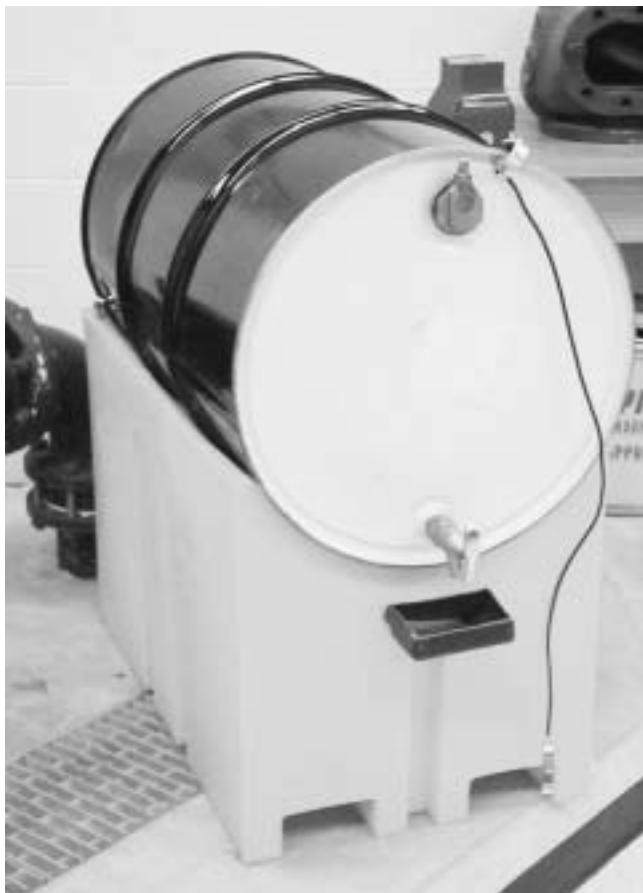
FIGURE 3.2 Typical flammable-liquids transferring arrangement
