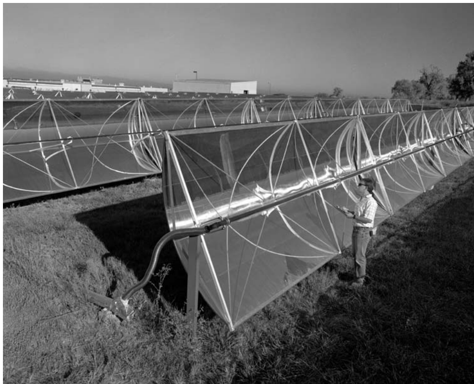
Figure 3.2. Parabolic trough solar collector for hot water heating at a prison in Adams County, Colorado.
