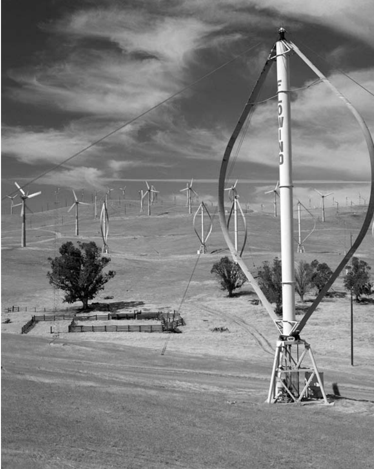
Figure 3.6. A Darrius-type vertical axis wind turbine.
