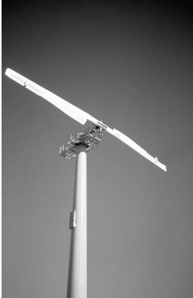
Figure 3.8. Two-bladed turbine at San Geronio Pass, California (250 kw).
