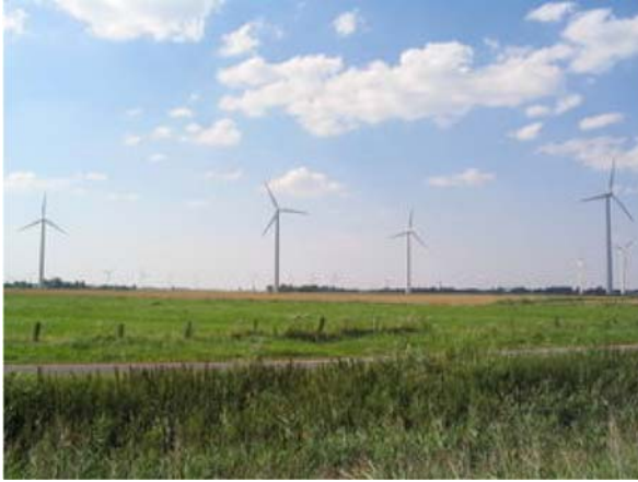
Fig. 11. Wind-driven farm in Neuenkirchen, Dithmarschen, Germany.
