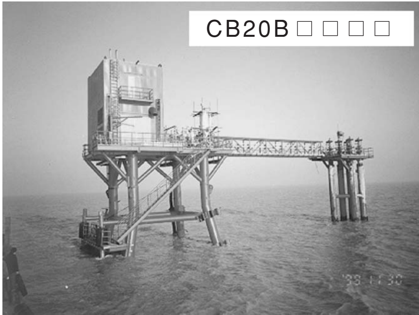
Figure 14.15 CB20B bucket foundation production platform developed for the Shengli Oilfield in China. It is the first one of its kind in China and went into production in October 1999
