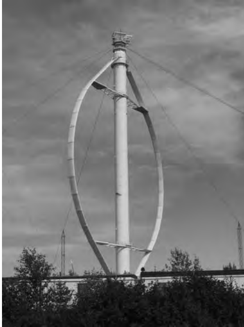
FIG 5.7 Typical vertical-axis wind turbine.
