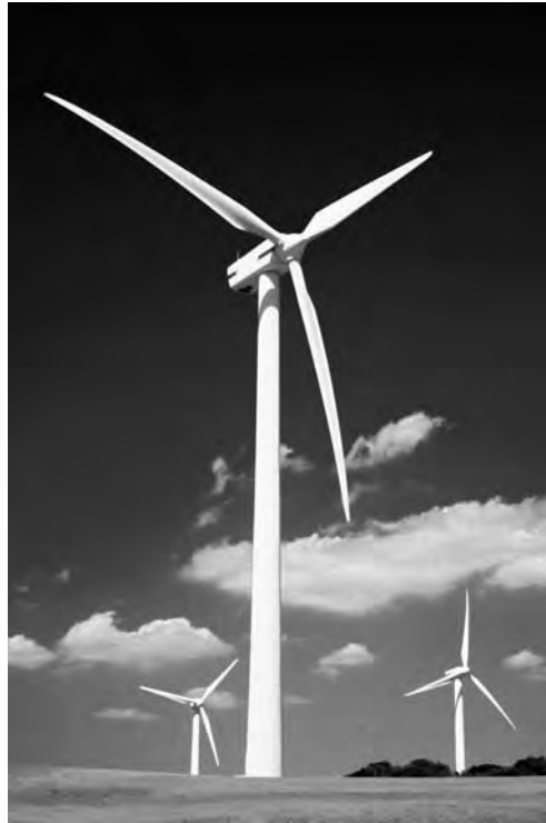
FIG 5.6 Typical commercial horizontal-axis wind turbine.
