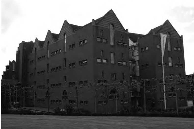
FIG 15.13 Queen's Building at De Montfort University, Leicester.
