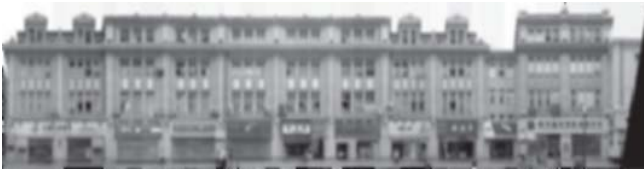
Fig.19 Whole facade texture
