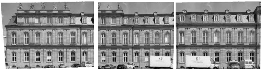
Fig. 16.3. Part of rectified images from Fig. 16.2.
