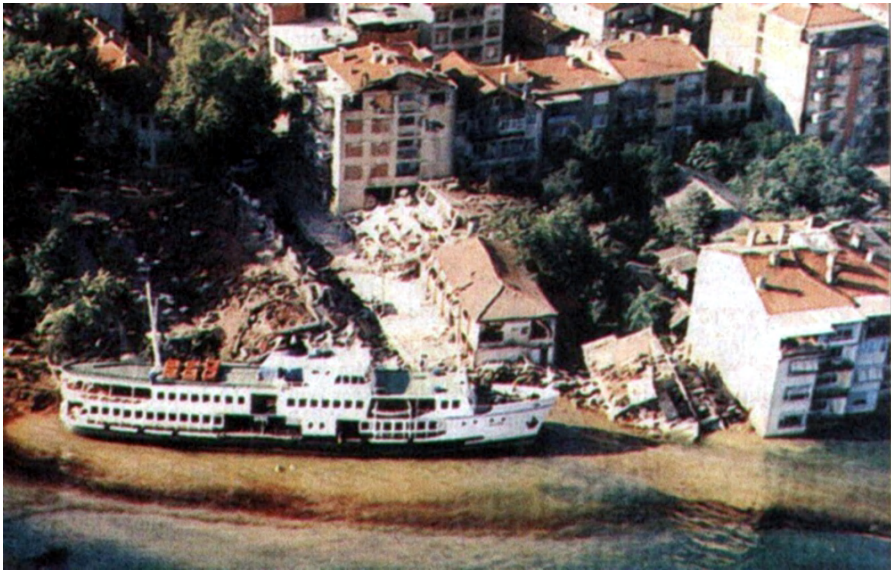
Fig. 1. Damage from the earthquake 1999, tectonic subsidence, ground liquification and the tsunami. The ship in the foreground thrown onshore by tsunami wave action. (Kandilli Observatory and Research Institute, www.drgeorgepc.com/Tsunami1999Turkey.html , accessed on 14.04.08)
