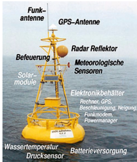
Fig. 4. Tsunami Sensors installed close to tectonic fault zones for detecting Tsunami waves when they start, ( http://www.forschung.bmbf.de/de/4879.php accessed on 18.04.08)
