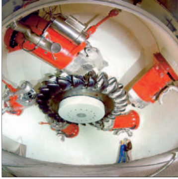
Fig. 2. Pelton turbine with five injectors (colorplate on p. 202).
