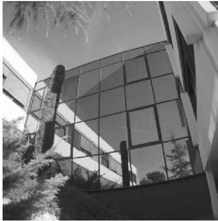
Figure 3.1. “Borel building” image (building from INRIA Sophia-Antipolis)
