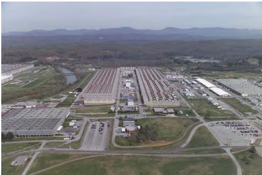
Fig. 8.5 The K-25 Gaseous Diffusion Plant at Oak Ridge, TN is no longer operational. This photograph conveys some sense of the extremely large scale of this operation (Photo credit. US Department of Energy and Knoxville News Sentinel, Oct. 17, 2004)
