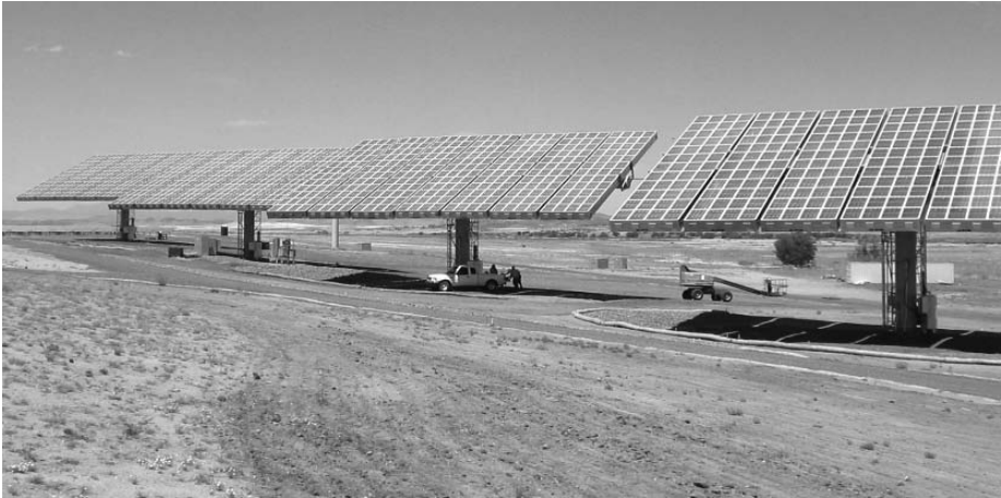
Fig. 1. Several 35-kilowatt (kW) CPV systems built by Amonix in Torrance, California, are installed at an Arizona Public Service power plant. The system uses Fresnel lenses to concentrate sunlight. The pickup truck in the shade gives an idea of size.
