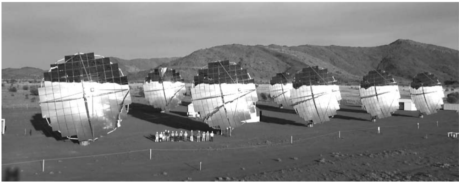
Fig. 2. Several 25-kW CPV systems built by Solar Systems in Hawthorn, Australia, and installed on aborigine lands. These systems use mirrors for concentration (see www.solarsystems.com.au ). Note the people in the foreground for an idea of size.
