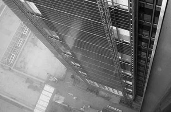
Figure 1.23 Dark blue solar panels in thin film Si undergoing integration on the façade of a 120 m tall skyscraper in Manchester. (Photo courtesy: Inhabitat.com).
