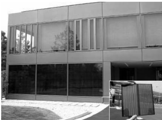
Figure 1.19 DSC-based modules coating the windows of the pavilion house of Toyota at Aichi's 2005 Expo. (Photo courtesy: Toyota).
