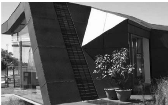
Figure 5.26 Built in 2005, this house in Australia uses the DSC-based Living Building Panel from Dyesol. (Photo courtesy: Dyesol).
