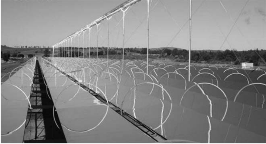
Figure 1.34 Flat reflectors move following the position of the sun and reflect the energy of the sunlight to the fixed pipe receiver above, where water is heated and becomes the steam needed to power a turbine. (Source: Ausra).
