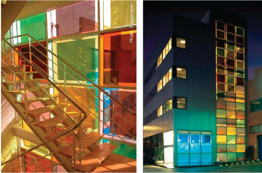
Figure 5.2 Example of indoor building integration of transparent colored DSC at the Schott Iberica building in Barcelona (Spain). (Photo courtesy: Dr. I. B. Hagemann and Schott Iberica).
