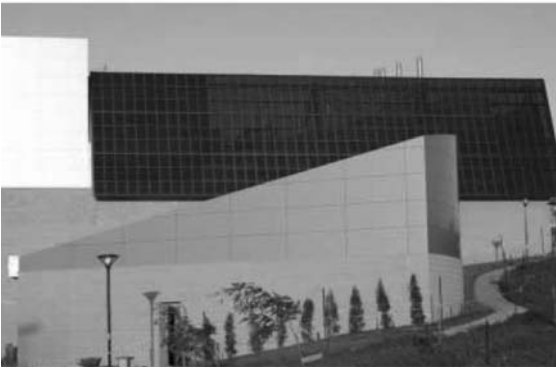
Figure 5.25 One of the facades of the new CSIRO Energy Centre, in Newcastle, Australia, was made with Dyesol's solar wall panels. (Photo courtesy of CSIRO and Dyesol).
