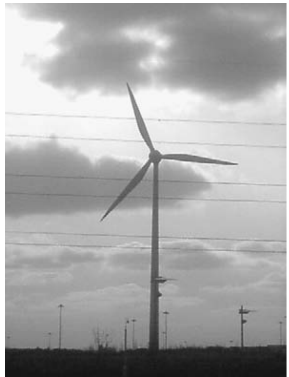
Figure 2-7 A wind turbine illustrating the power we can harness from the wind.
