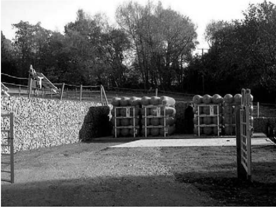
Figure 4-26 Hydrogen storage at the HARI project, West Beacon Farm. Image courtesy Dr Rupert Gammon.
