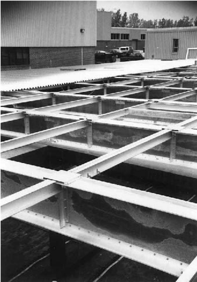
Figure 2.4 Water stains.
