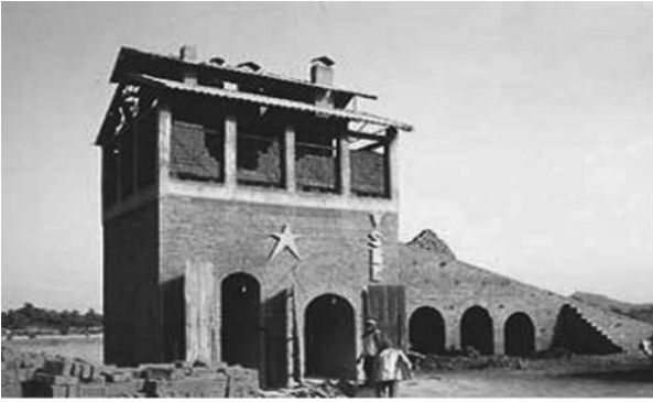
Figure 11.6. Two-shaft vertical shaft brick kiln at Varanasi, India.
