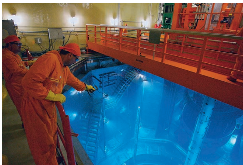
Figure 20.12 Refueling the core of a nuclear reactor.
