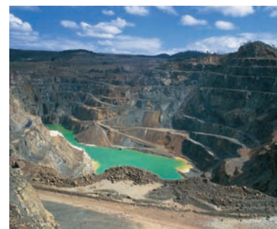
Figure 24.6 A cyanide pond for extracting gold from metal ore.
