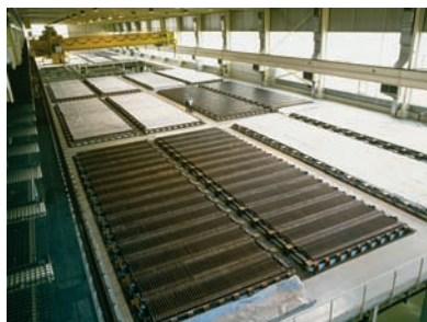
Figure 23.7 Copper cathodes used in the electrorefining process.
