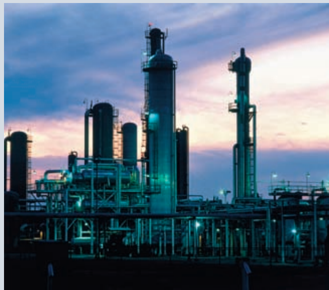
▲ Figure 13.21 Industrial distillation towers, in which the components of a volatile organic mixture are separated according to boiling-point range.
