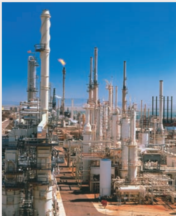
▲ Figure 25.9 Petroleum is separated into fractions by distillation and is subjected to catalytic cracking in a refinery, as shown here.
