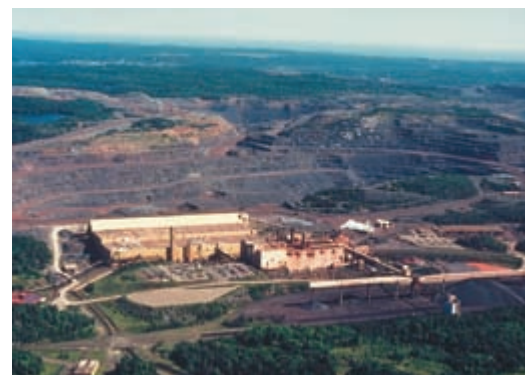
▲ Figure 23.3 At this open pit iron ore mine in Michigan's Upper Peninsula, crude ore is concentrated and formed into pellets suitable for shipment.
