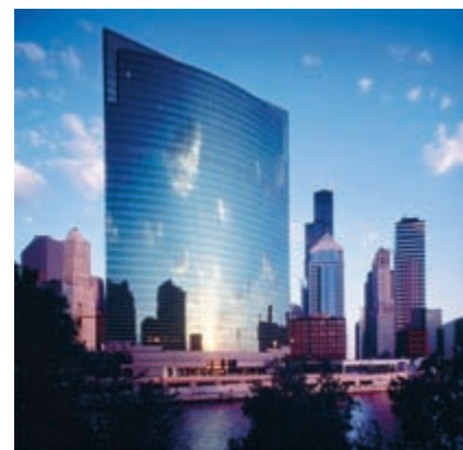
▲ Figure 12.31 The glass panels forming the outer walls of this building have a thin film of metal, which reflects a significant fraction of the outdoor light. The reflective glass provides privacy, reduces interior glare, and reduces the cooling load on the building in hot weather.
