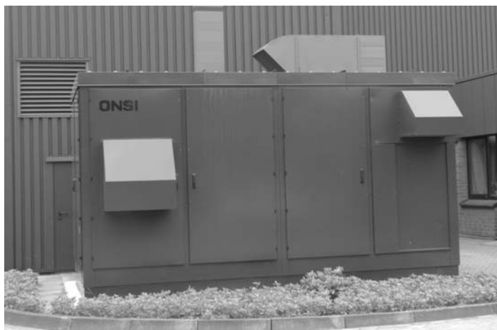
Fig. 5. Fuel cell for trigeneration at the St. Agnes Hospital in Bocholt
