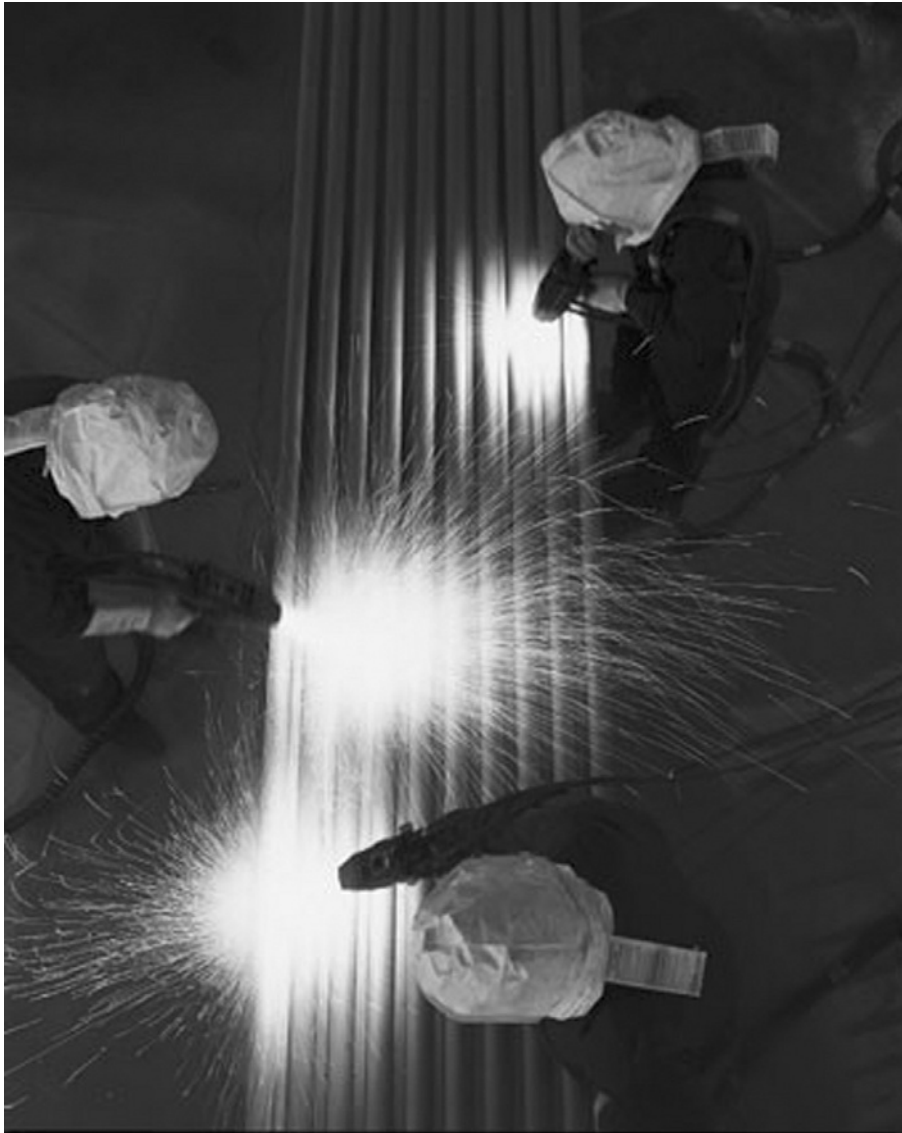
Figure 12.1-23 Thermal spraying, which is a variant of welding in some manifestations and of adhesive bonding or brazing in others, can be used for creating shapes as well as for applying coatings (as shown here). (Courtesy of Foster-Wheeler Corporation, Perryville/Clinton, NJ, with permission.)
