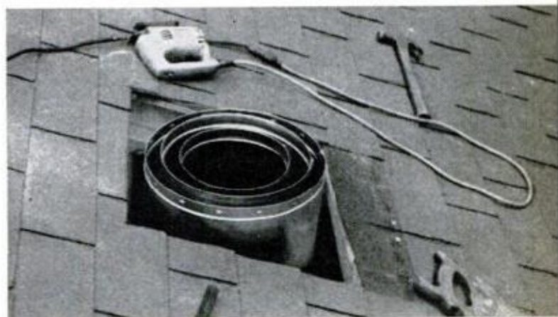
PACKAGED FIREPLACE (below) can be set on a wood floor, backed against a flammable wall with no fire hazard. Triple-pipe flue (above) is cooled by air
