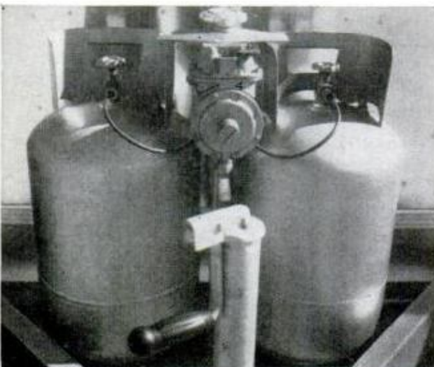
DOUBLE YOUR LP-GAS SUPPLY by adding a second gas bottle and installing switch-over valve connection
