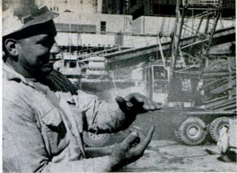
PILE DRIVER FOREMAN on San Francisco construction project uses this signal to tell crane operator to "hoist hook slowly." The operator's view of the hook is often obstructed. Television stage manager (below) uses a signal peculiar to the trade to warn news commentators that only half a minute is left in show
