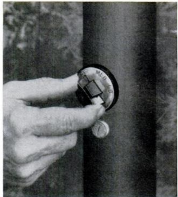
TO TURN ON GAS, valve is pressed inward, turned counterclockwise. Never light gas with cover closed
