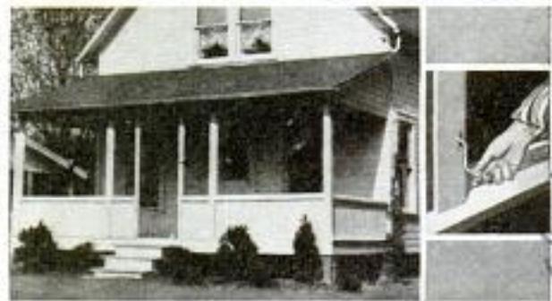
Open porch becomes an extra room when metal blinds, controlled by crank, lower right, are installed
