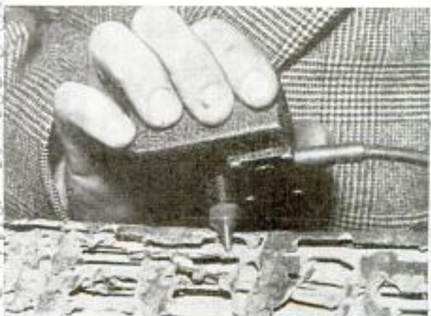
Radio detector amplifies sound of gnawing termites
