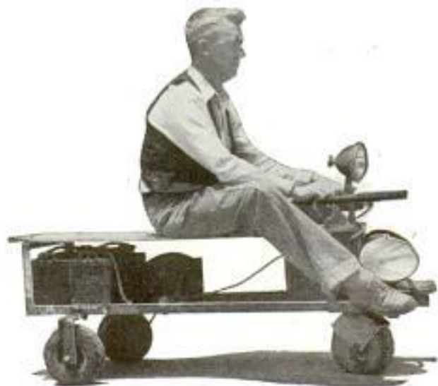
Electric three-wheeler for tunnel can haul three men
