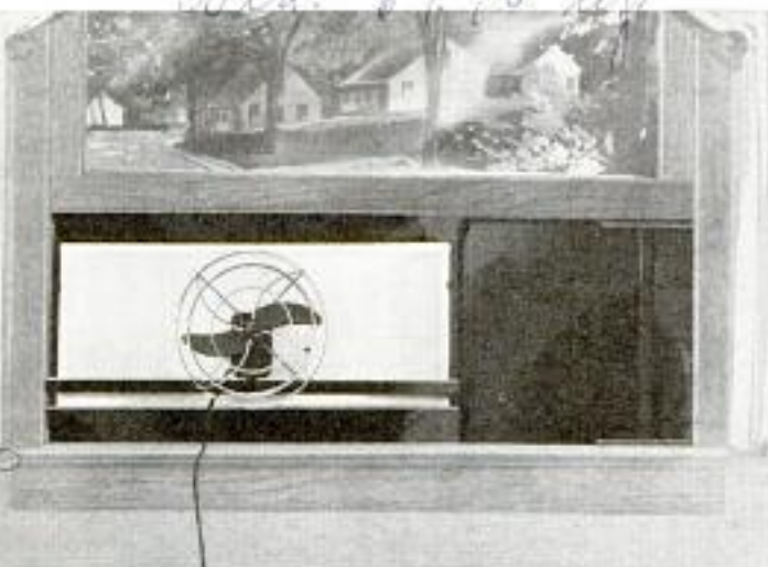
Moistened screen in window filters air and fan distributes it
