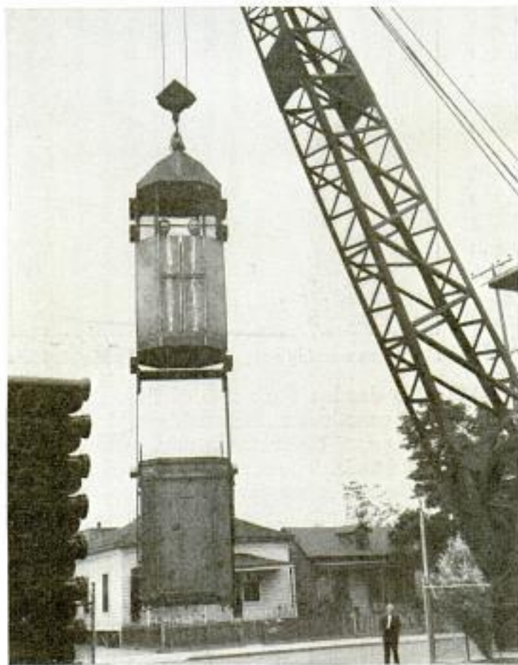
Giant crane lifts men in steel cage from aqueduct tunnel shaft
