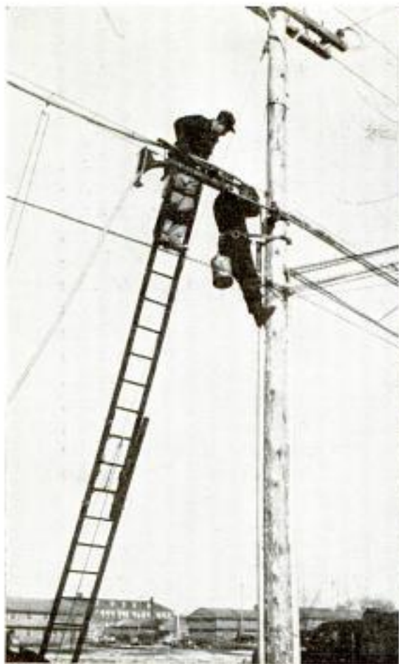
↑ Linemen pulling a 303-pair cable at a pole on Camp Custer reservation during a speedy installation job
