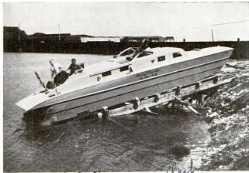
Sea sled designed for landing invasion troops slides down the rails to take its first dip
