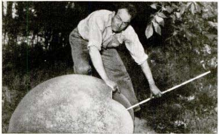
Balloon is inflated after pouring concrete over it, then allowed to set in the form of an igloo. Lower photograph shows the finished shelter
