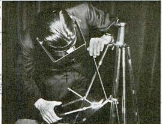
Top, electric welder produces either arc or flame from 110-volt line. Bottom, using it as flame torch
