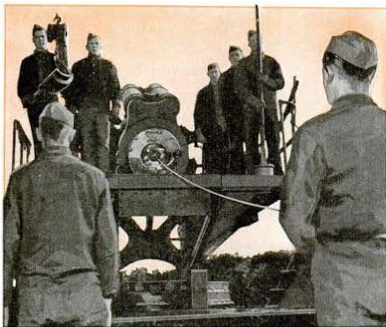
Ready to fire 8-inch railway gun which fires 260-pound projectile more than one and one-half miles, or a 200-pound projectile two miles
