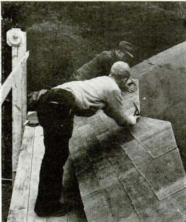
Covering a wide area, these strip shingles reduce the time needed to nail them on the roof, thus saving labor expense
