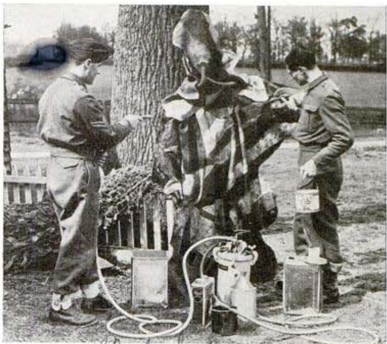
Using a brush and air gun to camouflage the loose-fitting drapery worn by a British soldier. This is nicknamed the army's "beauty parlor"
