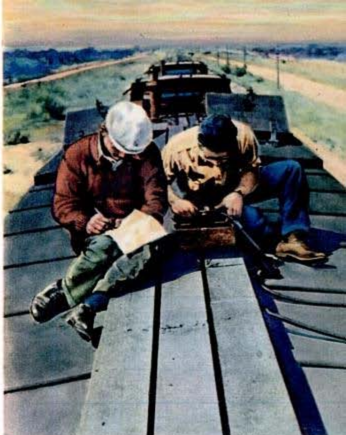
Arizona Engineers on roof of refrigerator car, above, are making temperature readings as train crosses desert. Below, Southern Pacific engine has its cab in front to give the crew better view around mountain curves mallet oil burner
