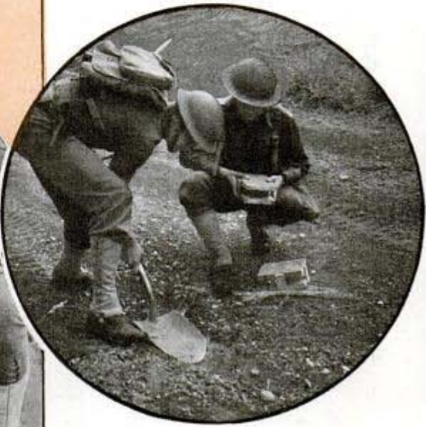
† Burying a land mine in a road. When a truck crushes it, smoke released from bottles shows the truck is out of action
