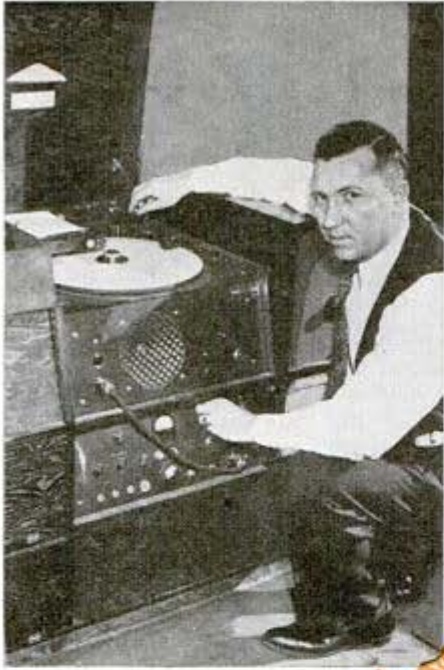
↑ Big recording phonograph "hears" every word that comes in and goes out of tower and makes a record of all orders
