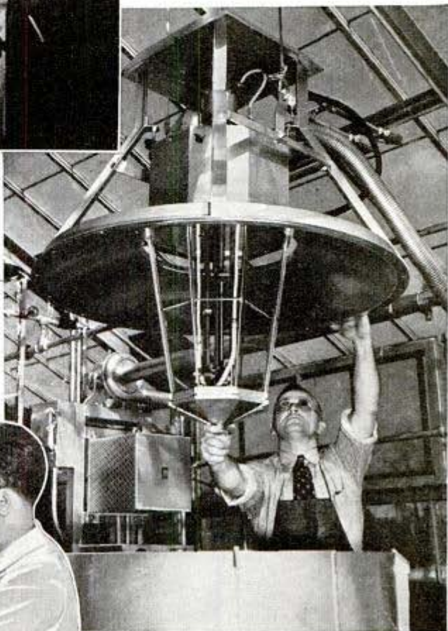
Carbon-arc lamp in greenhouse of pest-control laboratory is science's nearest approach to sun
