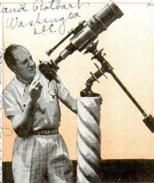
With an 8-millimeter Filmo camera equipped with 16-inch lens surmounted by telescopic rifle sight, this amateur shot "closeup" movies of the moon
