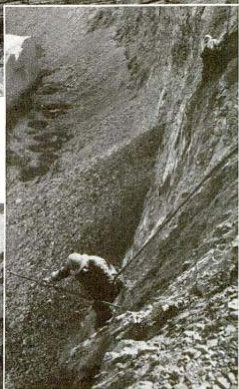
Photos by W. M. Rittase Above, miners trim the face of the pit after blasting. They use 5,000,000 pounds of dynamite a year. Left, the waste pile reminds visitors of Boulder Dam. Over a ton of waste must be dumped for every ton of ore mined. There are 36 working levels, rising 1,700 feet from pit bottom to mountain top.
