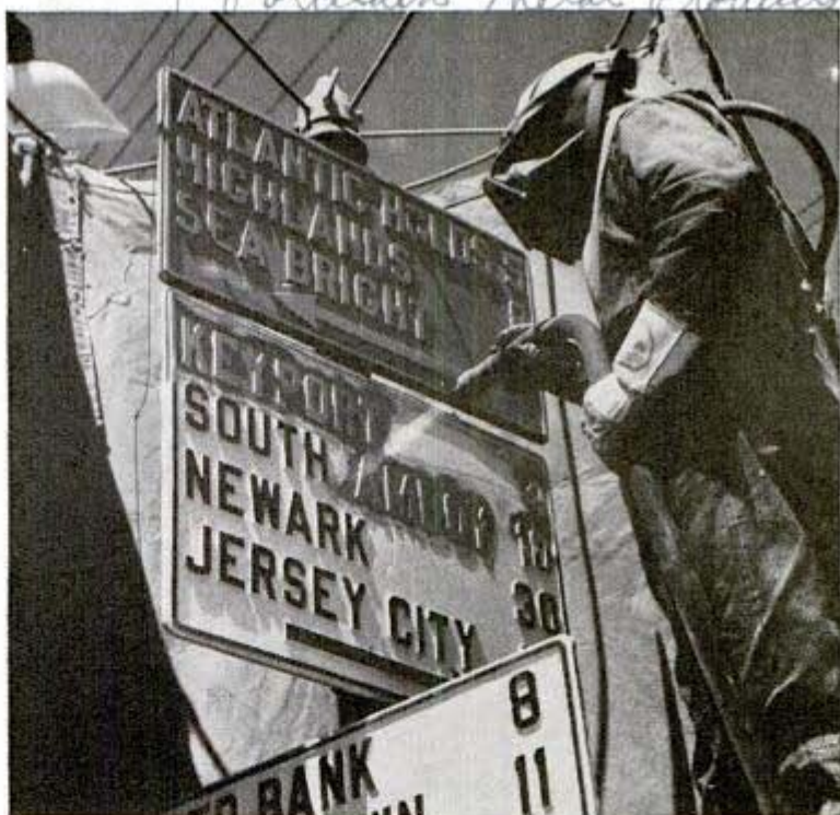
In less than 15 minutes the sand blaster removes all old paint from a New Jersey road marker. This is a regular "spring cleaning" routine. Below is a strip of the 160-mile Pennsylvania Turnpike and some typical road signs. The advice to "use both hands" is on a Missouri road
