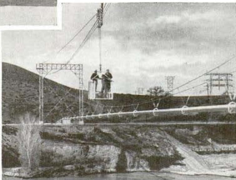
An emergency cable car ferries trouble shooters across a river, over a pipe line slung well above high water
