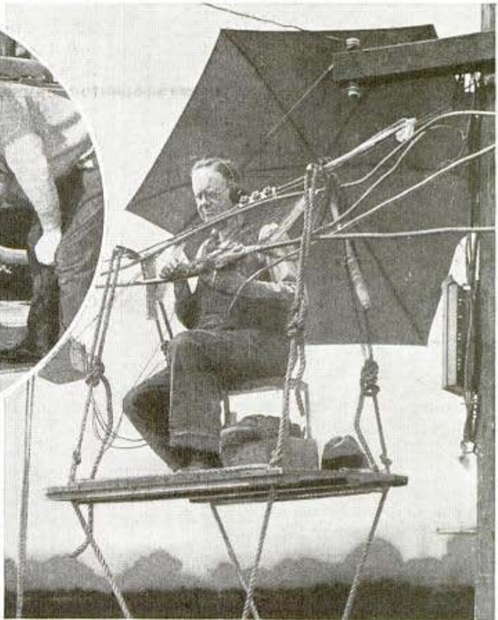
Working in a maze of wires, the power company trouble shooter can spot a faulty line immediately by employing his Wheatstone Bridge
