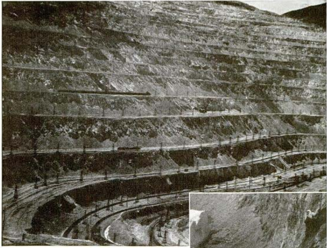
In the vast amphitheater of Bingham Canyon, west of Salt Lake City, is the largest open-pit copper mine in America, from which Utah Copper company moves 150,000 tons of ore and waste daily. Electric shovels load ore into what appear to be toy trains (above), but they run on standard-gauge electrified railway. There are nearly 100 miles of track on the level tracks, dump tracks and terraces
