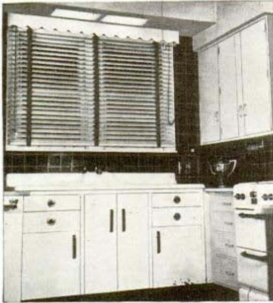
Cabinet-type sink sizes are: 14 x 20, 16 x 24, 18 x 18, 20 x 24, 20 x 30, 20 x 32, 18 x 42 and 22 x 48 inches. Last two are double sinks
