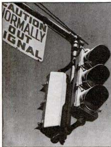
Lamp above is "normally out," letting main road traffic flow until car on side road lights it
