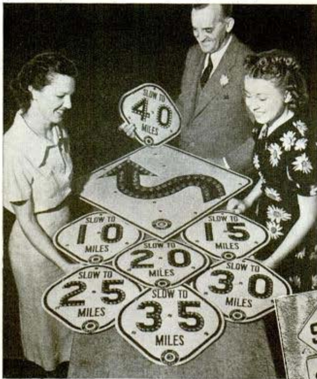
Top, a new type of "Slow to—" reflectorized warning signs that are now being installed along western routes Right, an assortment of familiar signs. The shapes of "Stop," "Slow" and regulatory signs are standardized Road to Ensenada, Mexico, from California border is outlined on map sign with distances in miles and kilometers
