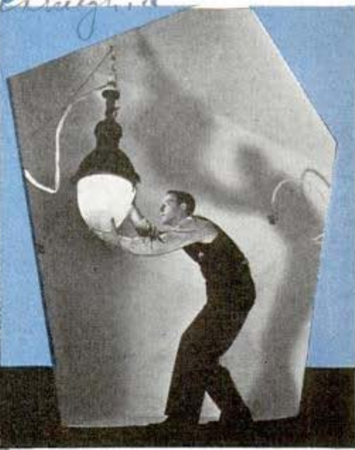
Engineer inside a 20-sided testing device equivalent to a 10-foot sphere which was built by Westinghouse illuminating experts Lamp div. Bloomfield, N.J.
