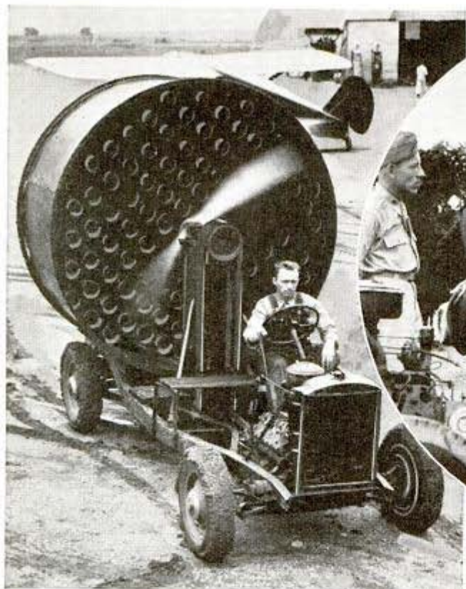
↑ Commander E. F. McDonald, Jr., inventor, points to five-belt pulley that transmits power from shaft of 85-horsepower engine to seven-foot propeller
