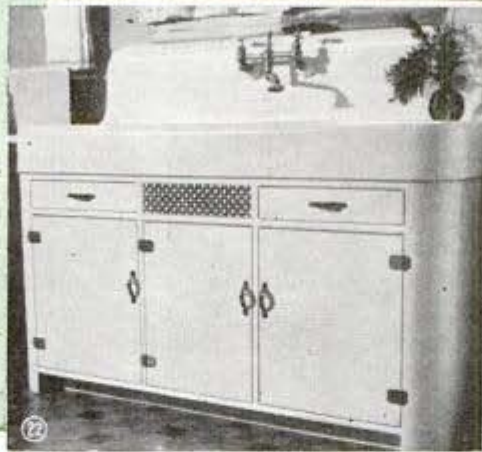
Often an old-model sink can be fitted with a cabinet as in Fig. 22, framework of which is shown in Fig. 21
