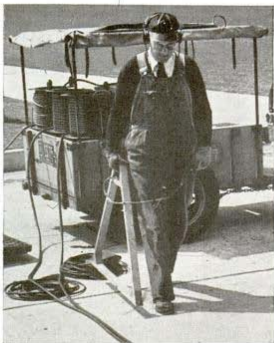
Above, hunting leaks in power line with a detector that sets up a buzz near the trouble site
