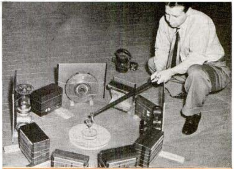
Using a tiny tube of radioactive yttrium to take pictures of steel, in search of hidden flaws
