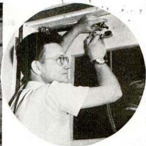
Flies buzz busily in the lethal chamber above until a scientist comes along with an air gun and shoots insecticides through the ports. Later the results are evaluated
