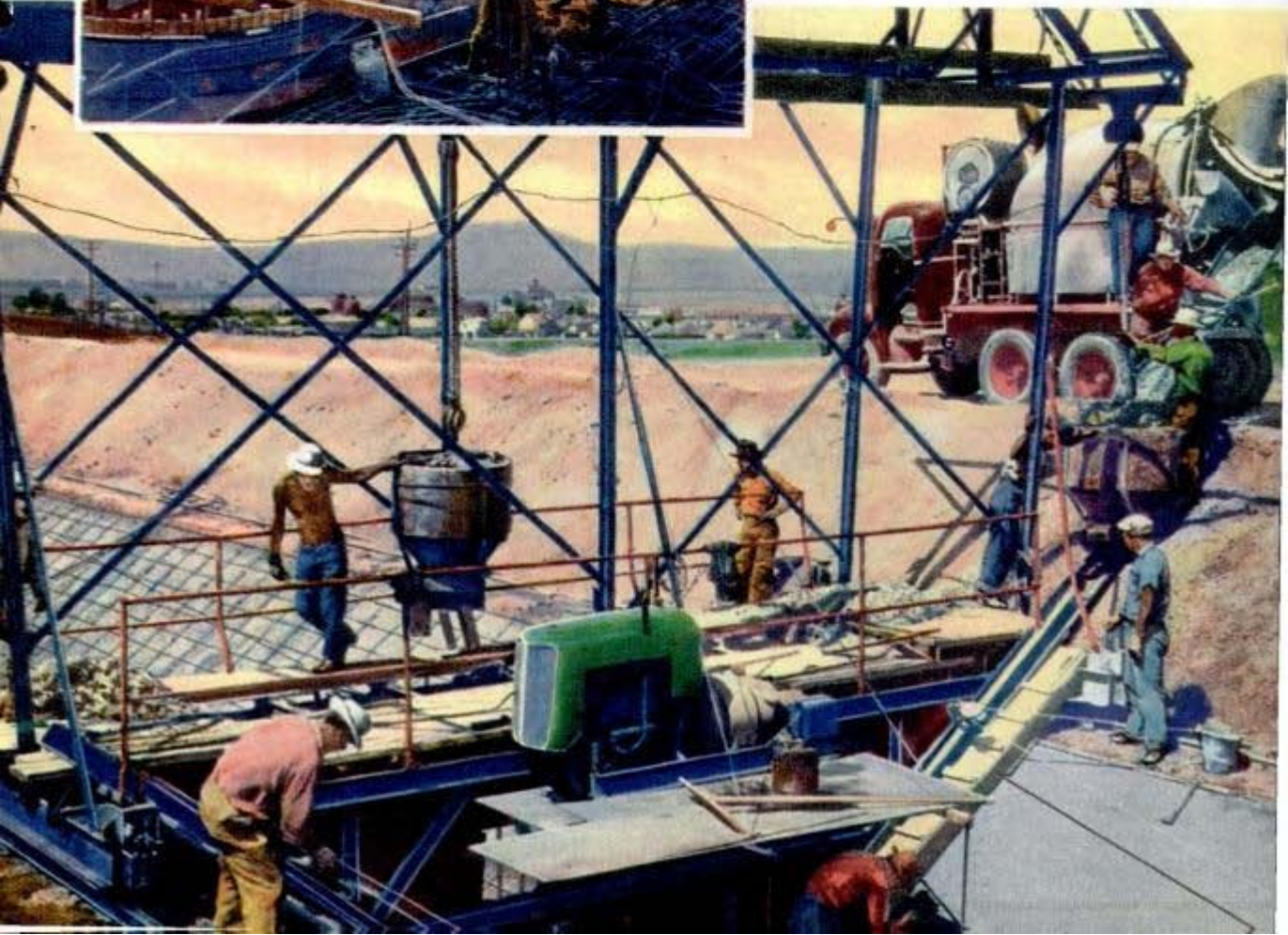
At left, pouring a four-yard bucket at Shasta Dam. Below, lining the Contra Costa canal with hot asphaltic concrete agitated in mixer
