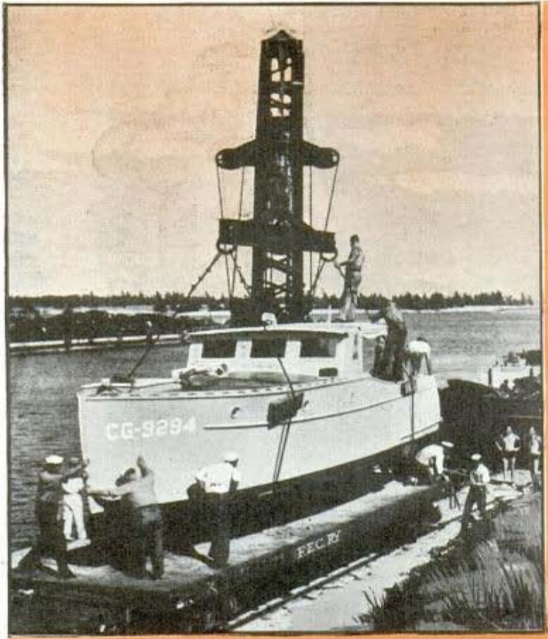
Even boats must travel by rail. Here a coast guard vessel is lifted aboard a Florida East Coast flatcar by a special crane
