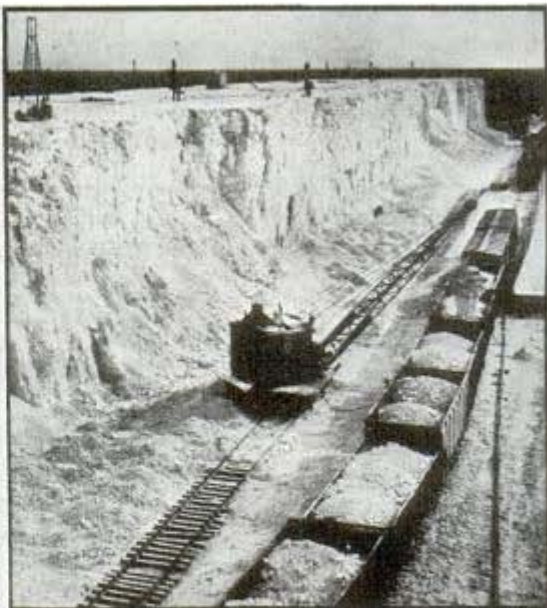
Above, storage pit of Freeport sulphur mine after molten sulphur has been pumped up. America produces plenty of sulphur
