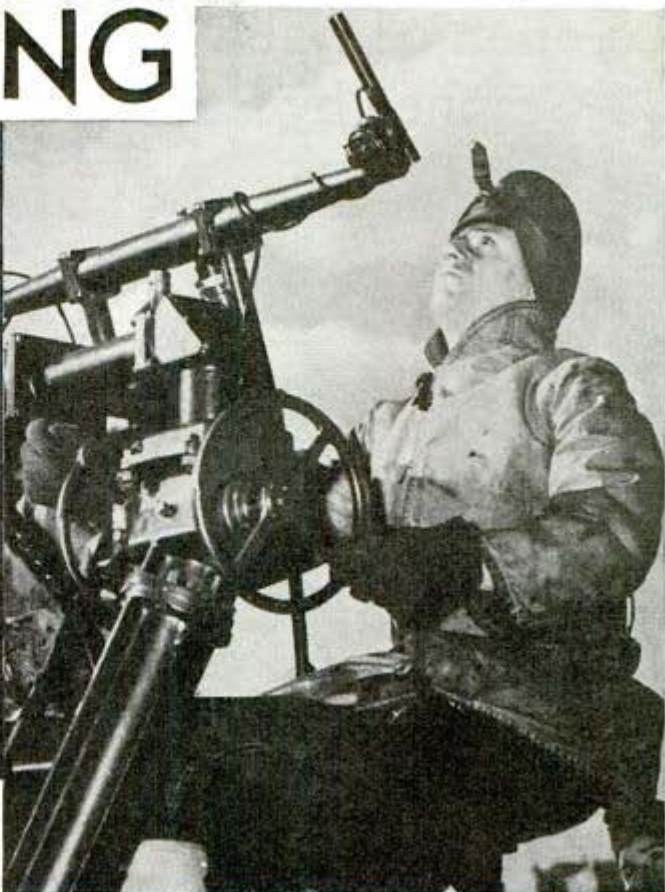
Lateral tracker, above, points weapon from side to side in azimuth, keeping the sight continually on the target
