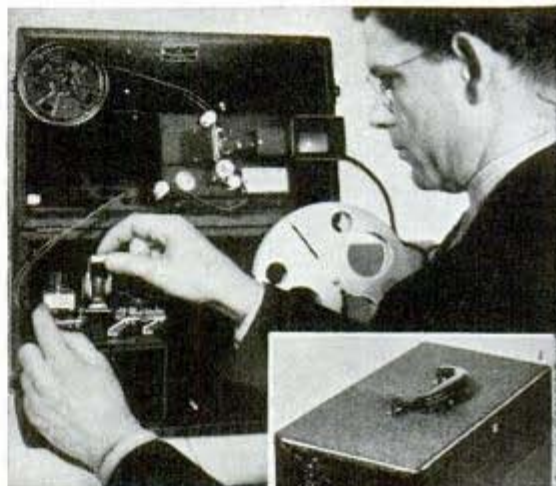
Movie film viewing and editing set is ready for work as soon as case is opened. Inset, it closes compactly
