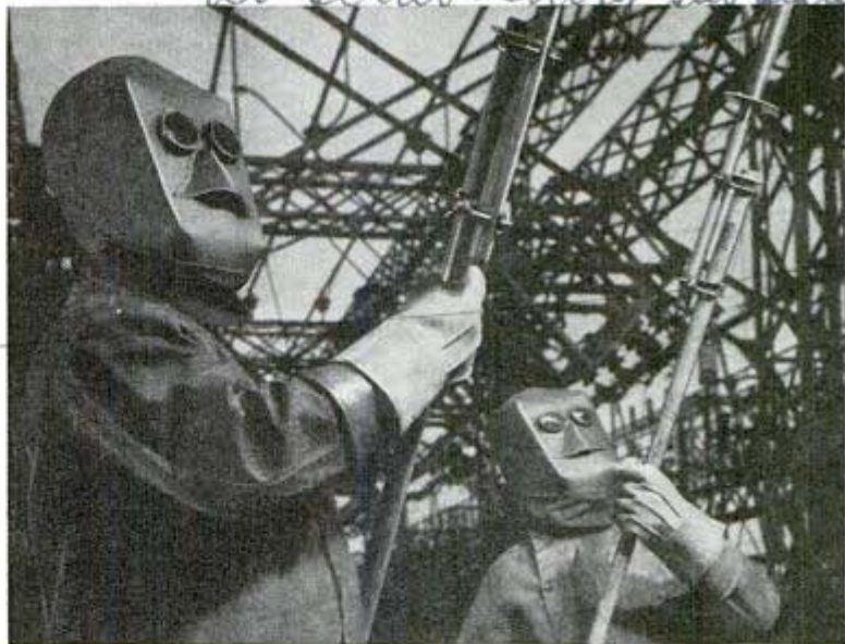
Though accidents are rare, danger always lurks around power stations, so these men take precaution by wearing heavily insulated hoods and clothes
