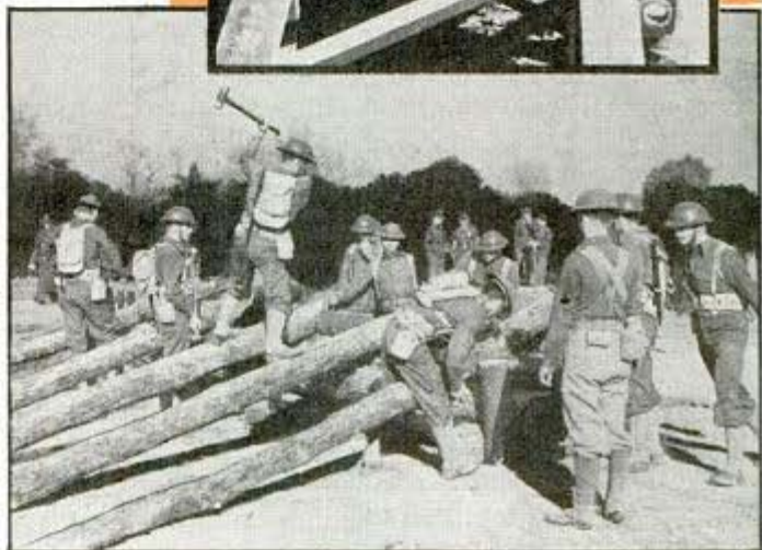
Right, more practice for the engineers—constructing a log barrier in the path of "enemy" vehicles
