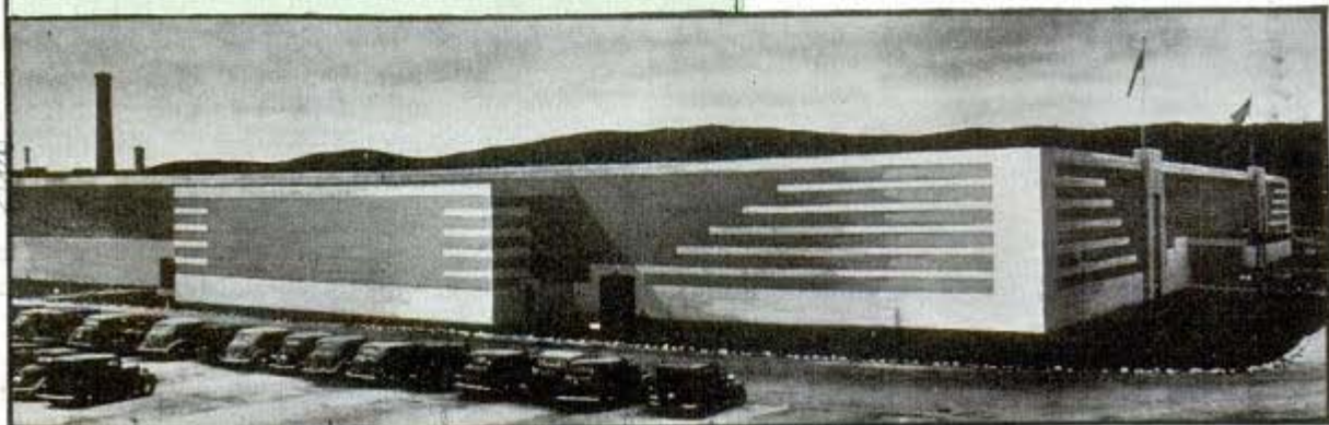
Above, an air-raid shelter being studied by U. S. housing officials. Below, a windowless factory that sets a standard for "blackout" plants with fluorescent lighting
