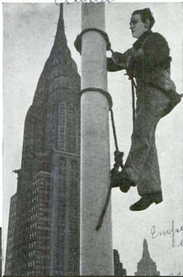
Andy Collins Above, climbing a 75-foot flagpole by inching up first the top rope, then the lower. Below, nearing the bottom after the day's work; what appears to be steps is really a series of cornices supporting the tall flagstaff
