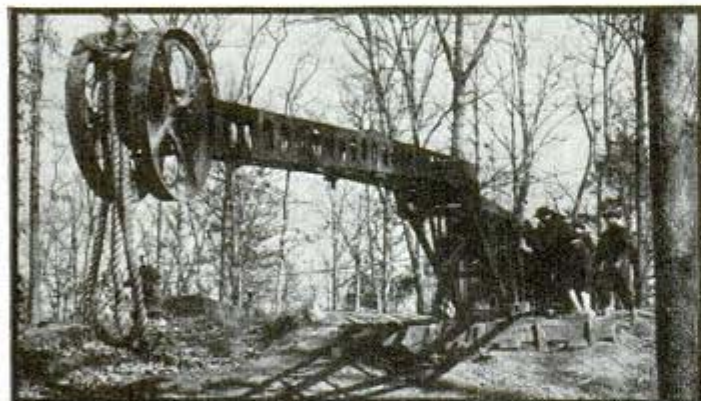
Chub. Army engineers preparing to cross river in assault boat. Below, first stage in the construction of a portable steel bridge. Recently the engineers erected a 10-ton span in 75 minutes
