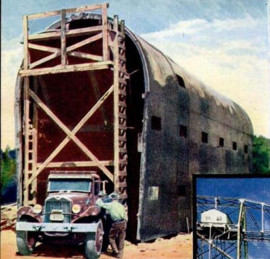
Portable wall and arch form at left is used in concreting tunnels on railroad relocation around Shasta reservoir; concrete is poured through windows from inside to form foot-thick walls and roof. Below, the downstream face of Friant Dam, from Fresno county abutment. Across bottom of pages is a sketch of the entire Central Valley project of California
