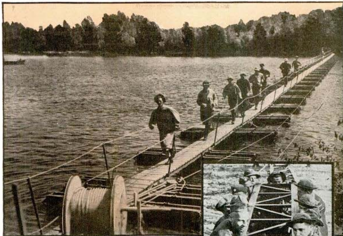
Above, crossing footbridge which engineers erected in quick time. Right, joining sections of steel bridge in demonstration of speed with which engineers work
