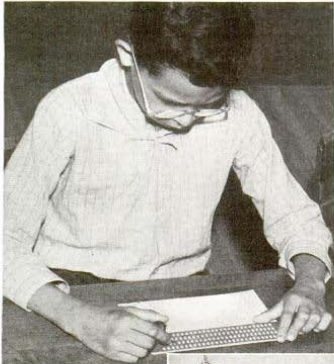
Above, Braille slate and stylus enable almost blind boy to write quickly without strain on his eyes
