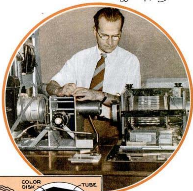
Above, Dr. Goldmark, CBS engineer, at still projector of color television equipment which he developed. Left, sketch of how color television works. The setup is identical with black-and-white television, save that color disks are used at transmitting and receiving ends and that controls include color mixer.
