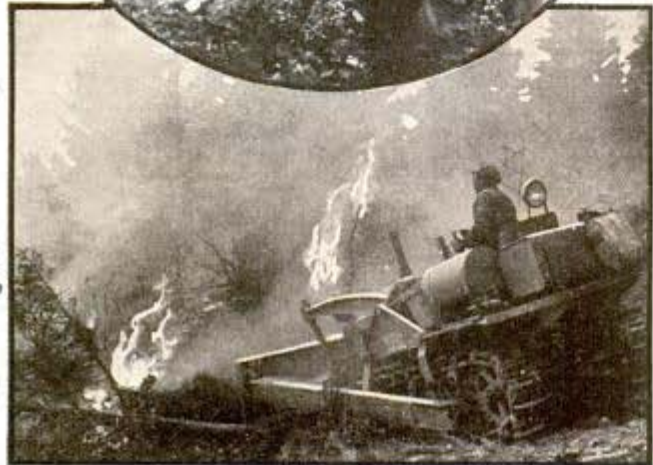
Big bulldozer at left, with angled blade like a snowplow, outdoes 100 men digging trenches and throwing dirt on flames
