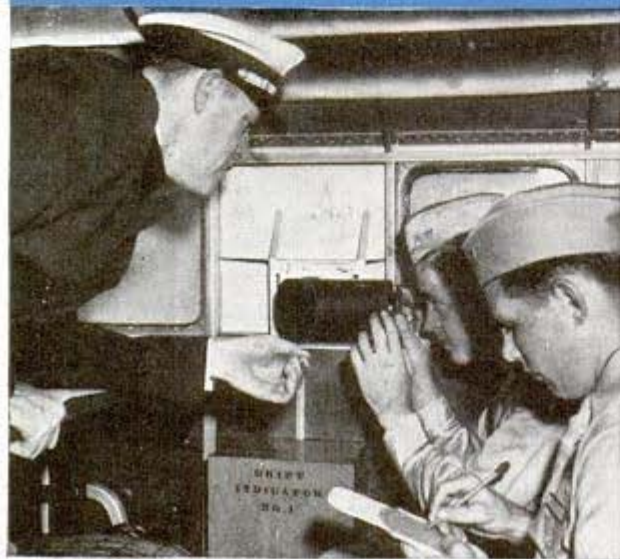
Above, two U. S. Army students watch instructor plot course in "flying classroom." Below, instructor aiding student using the drift indicator
