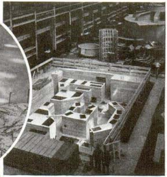
Circle, giant "nails"—steel piles driven down twenty-nine feet and filled with concrete so each could support thirty tons. Right, twenty-four ton "chair of concrete on which 350-ton boring mill has been installed. Below, installing mighty cutting tool
