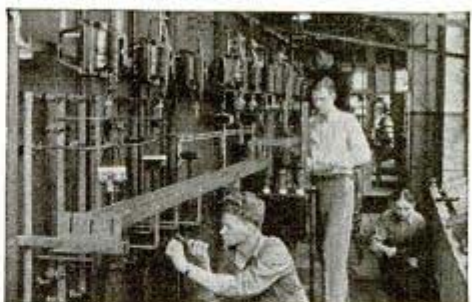
A Real Switchboard in the Coyne Shops
