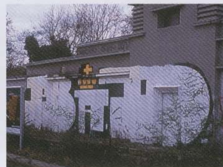
Bad – Treptower Park
