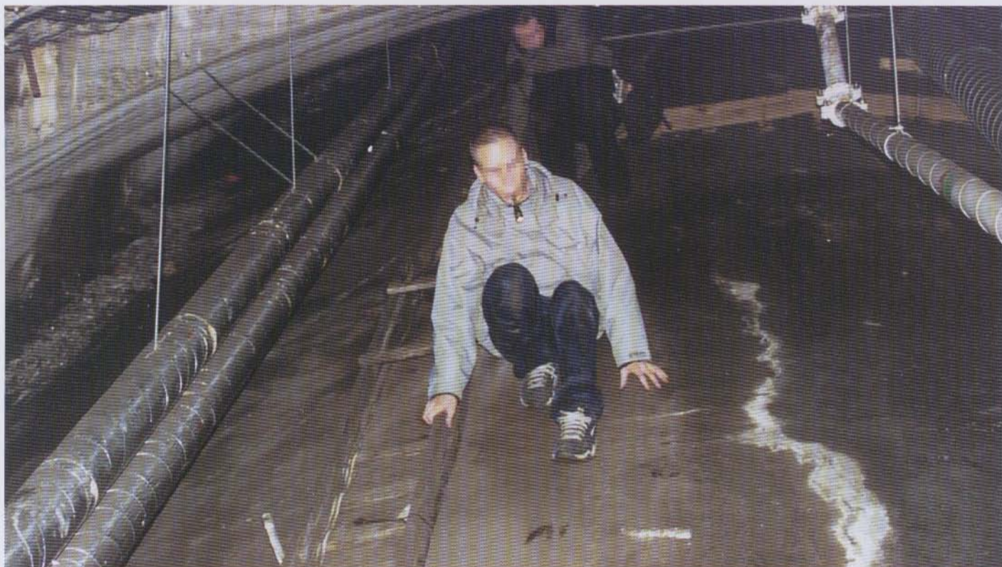
In the subway tunnels.
