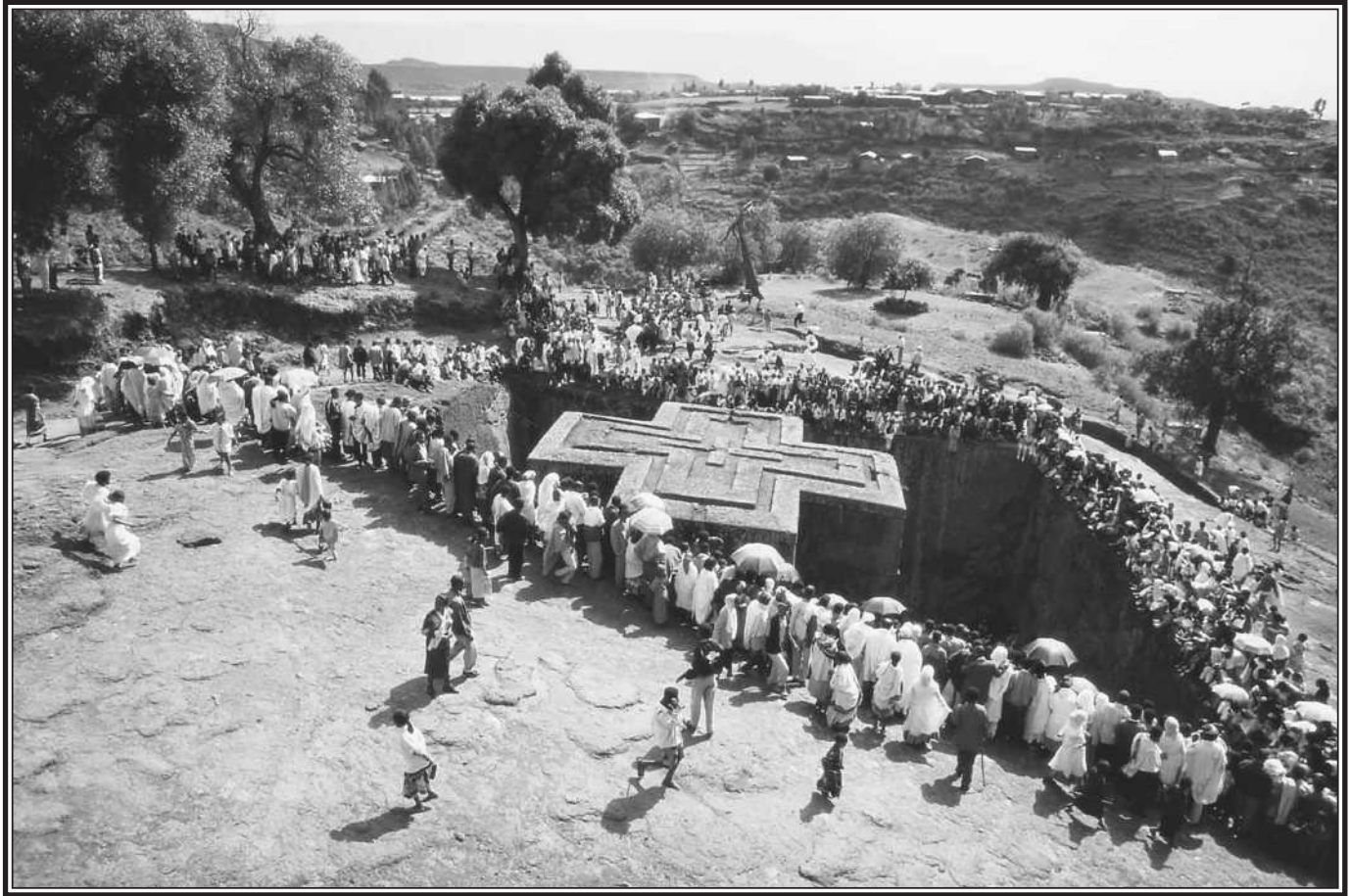
The stone church of St. George in Lalibela, Ethiopia, is more than 700 years old. Designed in the form of a cross, it was cut from the surrounding rock.
